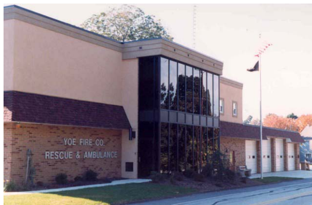
Station 36 - Yoe Borough
